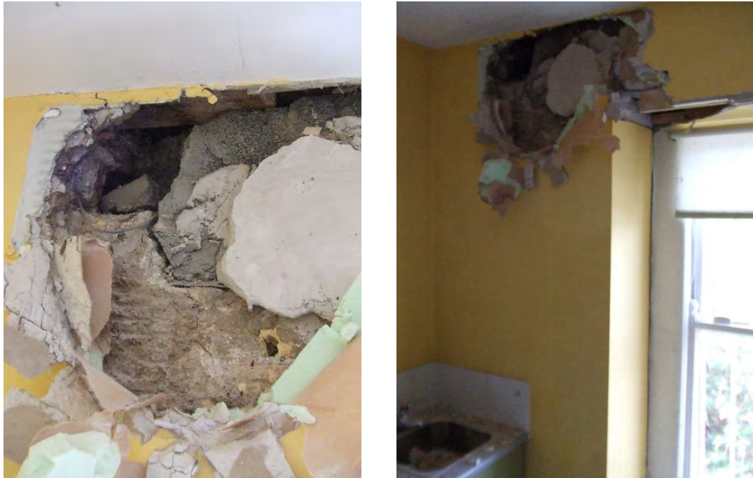
Figure 3-4: Photos of Internal Investigation
